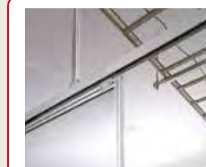
Hanging sliding doors with an opening of 2 m supported by upper and lower frames.
